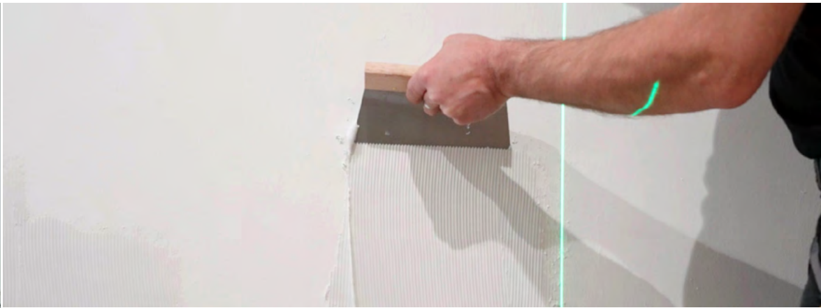
Tecnografica Showroom, Castellarano Installation process of Lamiera Fiammata design on Ultralight slabs
